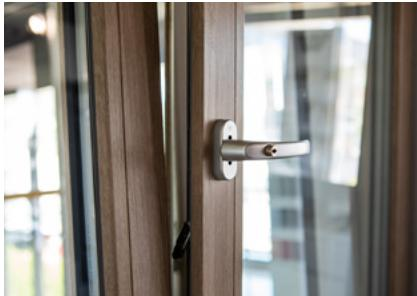
This solution is aimed at locking the leaf in the tilted position after rotating the handle by 90 degrees to the horizontal position, which prevents the leaf from moving from the tilted to the open position. Only after the handle is unlocked with a key can the window be opened. This solution provides safety for children and at the same time makes it possible to ventilate the room with the window tilted.
