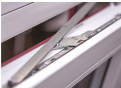
Problem-free operation of the window, primarily when windows are difficult to access, thanks to the handle in the bottom part of the window leaf. The comfort scissor stay can only be used in the RU window version, it cannot be used with concealed hinges.
