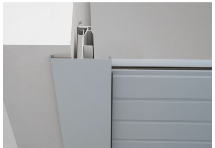
Installation in the opening – fascia panel in front of the opening
