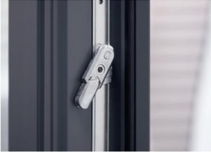
Drive gear with a handle rotation lock and a leaf lifter
